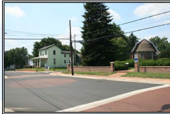
Intersection of Main and Walnut Streets
