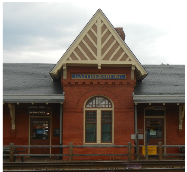
The Gaithersburg B&O Railroad Station was built circa 1884.
