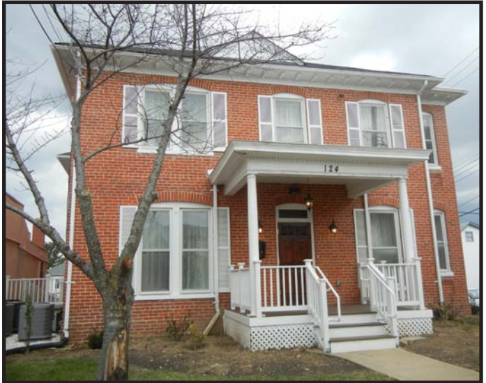
HD 15 - Exchange Building
