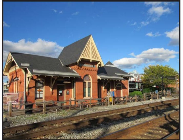
HD 3 - B&O Railroad Station and Freight Shed
