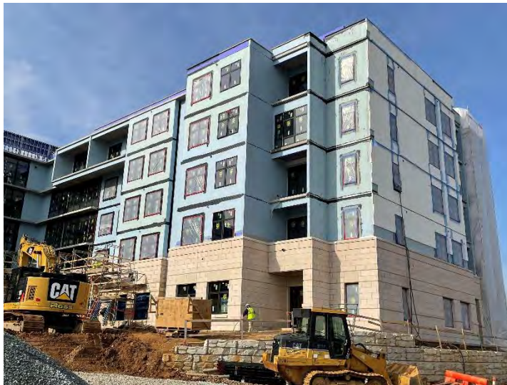
The Carnegie, a new senior housing project under construction
