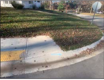
A City sidewalk does not continue onto the adjoining block.
