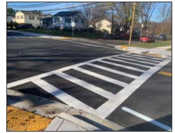
A “zebra” style crosswalk with a curb extension, such as this one crossing Baltimore Road at Woodburn Road, is more visible to motorists than traditional crosswalks. Photo credit: City of Rockville.
